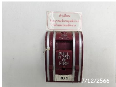
Fire Alarm Manual Station
