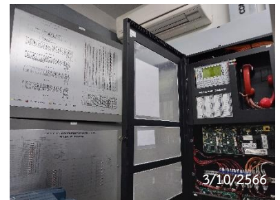
Fire Alarm Control Panel
