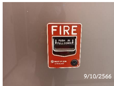
Fire Alarm Manual Station
