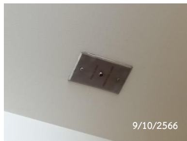
Fire Alarm Indicator Lamp
