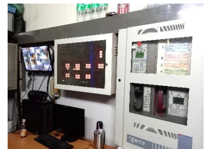
Graphic Annunciator Fire Alarm System
