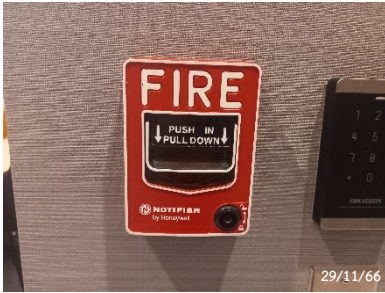
Fire Alarm Manual Station
