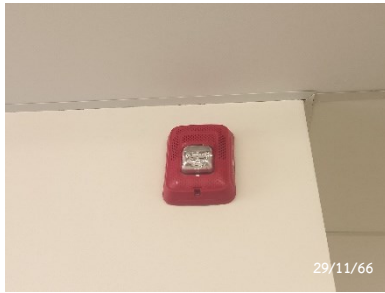
Indoor Selectable Output Speaker
