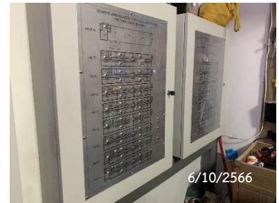
Graphic Annunciator Fire Alarm System
