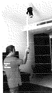
FLOOR 12 ROOM 1212 SERVICE TEST SMOKE DETECTOR ...NORMAL
