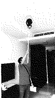
FLOOR 22 ROOM 2212 SERVICE TEST SMOKE DETECTOR
