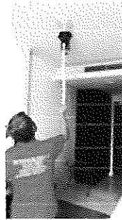
FLOOR 8 ROOM 804 SERVICE TEST SMOKE DETECTOR ...NORMAL
