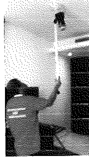
FLOOR 19 ROOM 1910 SERVICE TEST SMOKE DETECTOR ...NORMAL
