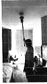
FLOOR 14 ROOM 1412 SERVICE TEST SMOKE DETECTOR ...NORMAL
