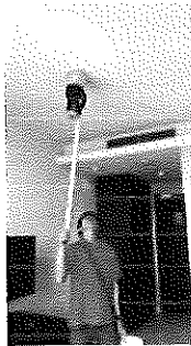
FLOOR 11 ROOM 1106 SERVICE TEST SMOKE DETECTOR ...NORMAL
