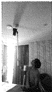
FLOOR 8 ROOM 808 SERVICE TEST SMOKE DETECTOR
