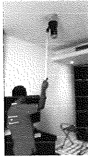
FLOOR 11 ROOM 1108 SERVICE TEST SMOKE DETECTOR ...NORMAL
