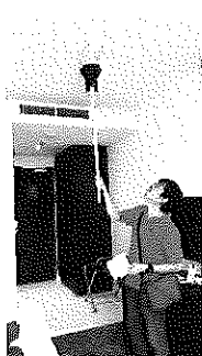
FLOOR 19 ROOM 1907 SERVICE TEST SMOKE DETECTOR
