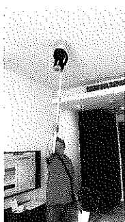
FLOOR 20 ROOM 2005 SERVICE TEST SMOKE DETECTOR
