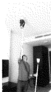
FLOOR 17 ROOM 1717 SERVICE TEST SMOKE DETECTOR
