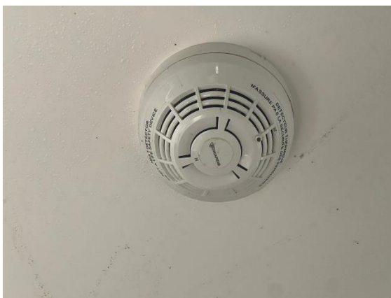
Rate of Rise Heat Detector
