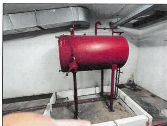
Diesel Fuel Tank of Fire pump
