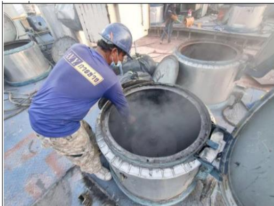
Picture 126 : Cleaning support insulator
