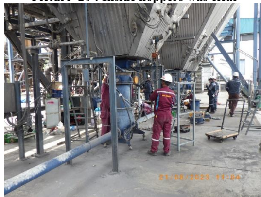
Picture 22 : Rotary valve below hopper
