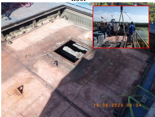
Picture 102 : Cut hot roof and lifted to the ground floor
