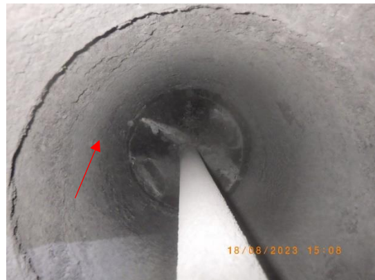
Picture 15 : Dust on inner support insulator surface
