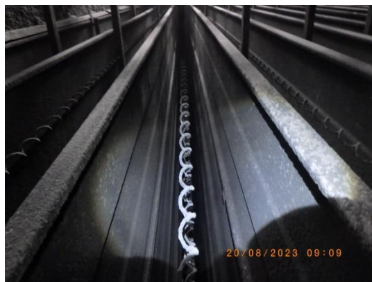
Picture 44 : All DEs were seen in tolerable tension
