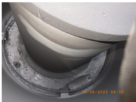
Picture 16 : Dust coating on outer support insulator surface
