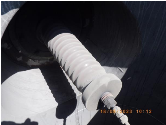
Picture 73 : Dust accumulated on lead-in insulator surface
