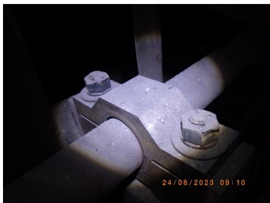
Picture 122 : Replaced DE horizontal bearing
