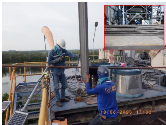
Picture 104 : Dismantled old CE and cut on the ground
