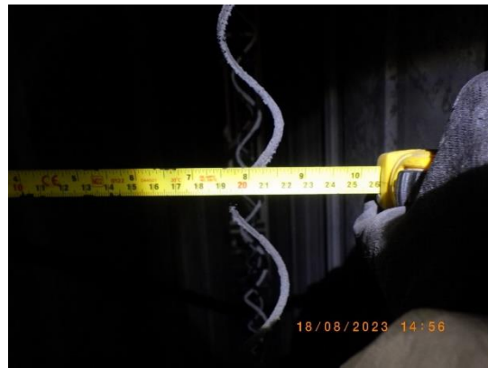
Picture 30 : All DEs were seen in tolerable tension and gap between CE-DE were normal
