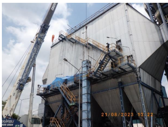
Picture 96 : Lifting CE box to vertical position
