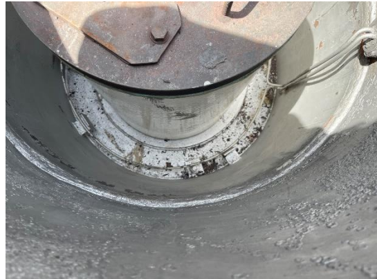
Picture 127 : Cleaned support insulator
