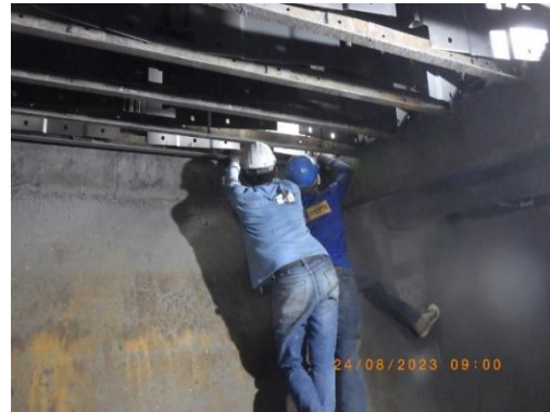
Picture 109 : Installed rapping bar bolt nut
