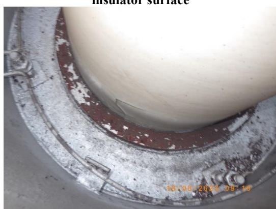
Picture 18 : Cracked support insulator
