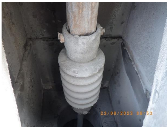
Picture 65: DE rapping insulator in low position and dust accumulated on surface
