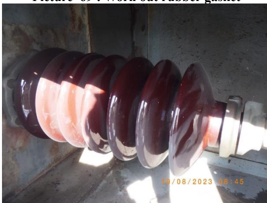
Picture 71 : Dust coating on HV-Bushing
