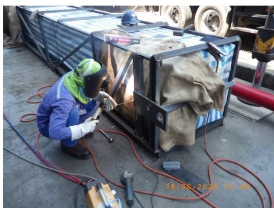
Picture 94 : Reinforcing CE box
