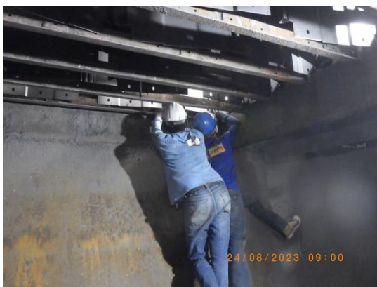
Picture 37 : CE rapping bar was intact
