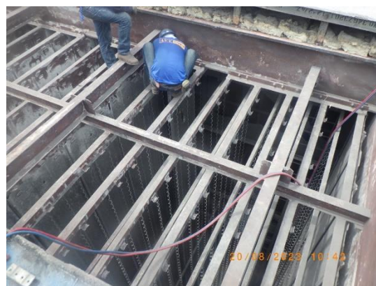
Picture 38 : CE suspension was intact
