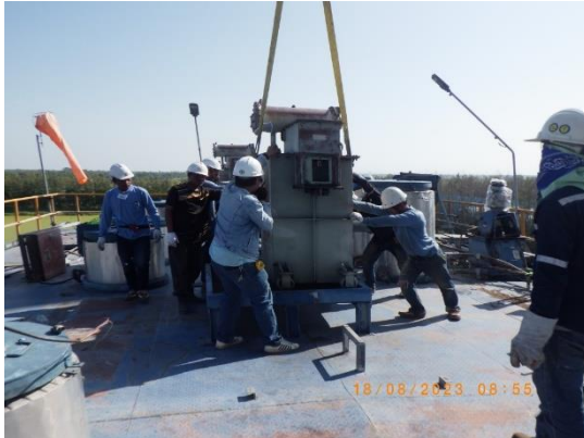
Picture 98 : Removing TR set
