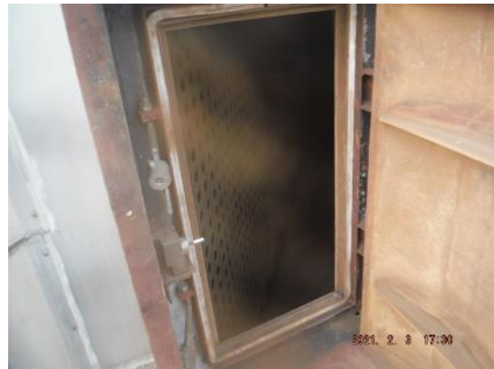
Sample 2: Example of silicone gasket installation on the access door
