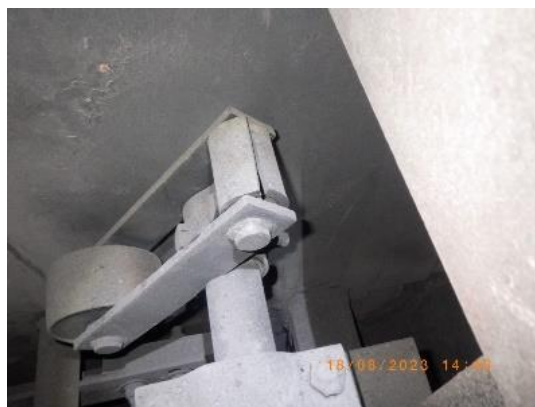
Picture 27 : Loosen CE hammer clamp bolt/nut
