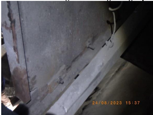
Picture 110 : Tack weld at CE bottom bolt nut
