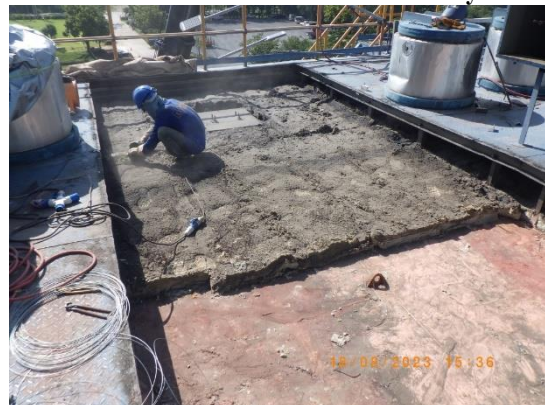
Picture 101 : Removing insulation
