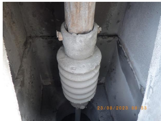
Picture 36 : Dust coating on rapping insulator
