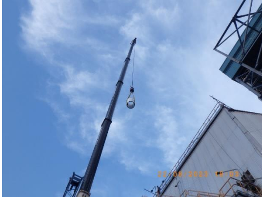
Picture 124 : Lifting support insulator to the roof
