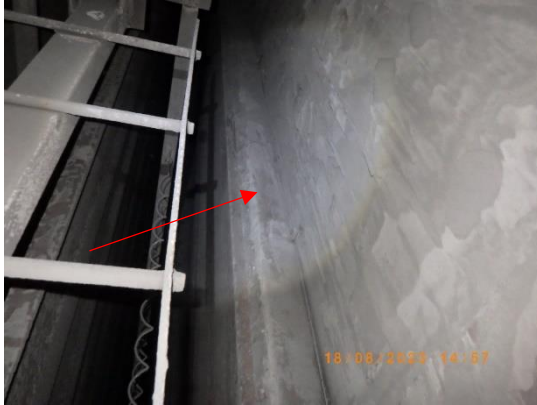
Picture 13 : Side baffle plate in normal condition
