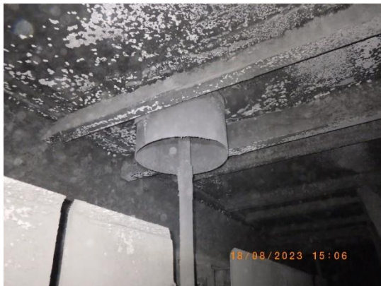
Picture 14 : Dust built up on protection conduit
