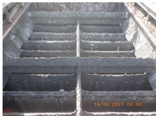
Picture 103 : Hot roof was dismantled
