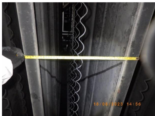
Picture 23 : CE still straight and gap between CE-CE were normal
