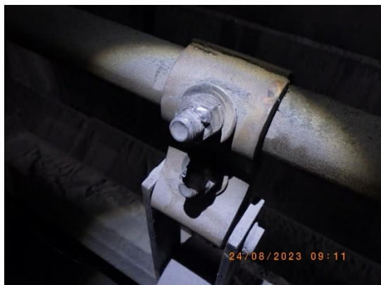
Picture 120 : Replaced CE hammer bolt/nut
