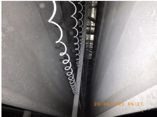
Picture 59 : DE frame still straight and contain DE with secure hook
