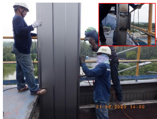
Picture 107 : Welding on CE interlock
