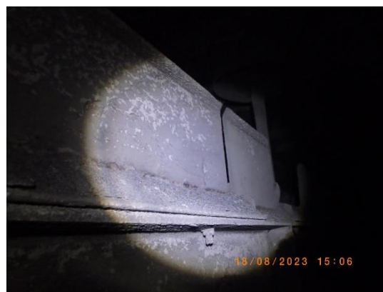
Picture 12 : Top baffle plate in normal condition
