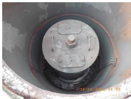
Picture 17 : Dust accumulated in support insulator chamber
