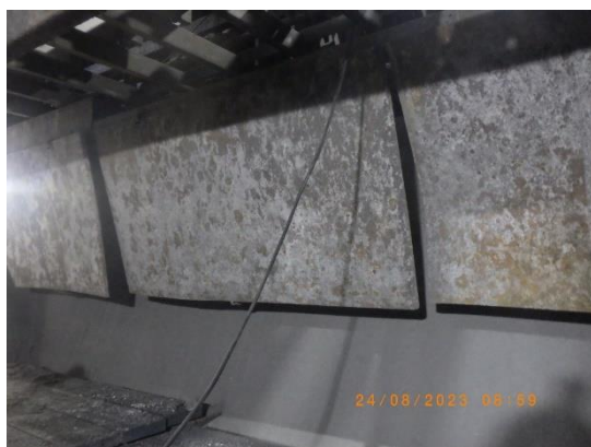
Picture 11 : Bottom baffle plate was intact
