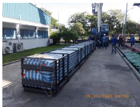
Picture 95 : Preparing CE box for vertical lifting
