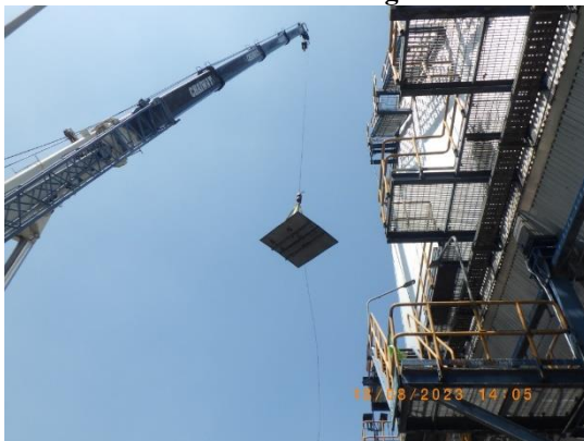
Picture 100 : Lifting cold roof to the ground floor
