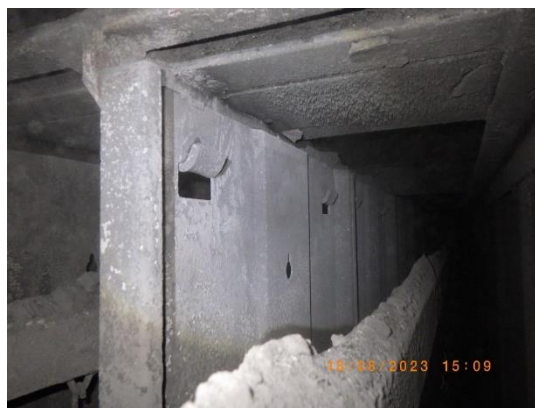
Picture 24 : CE suspension hanger were intact
