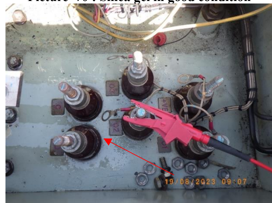
Picture 72 : Oil leakage from LV bushing
