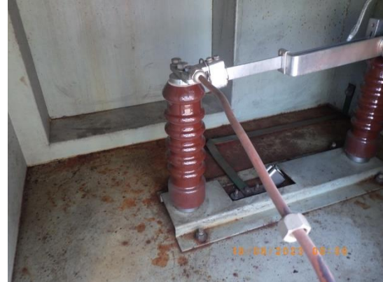
Picture 68 : HV compartment casing has corroded inner surface
