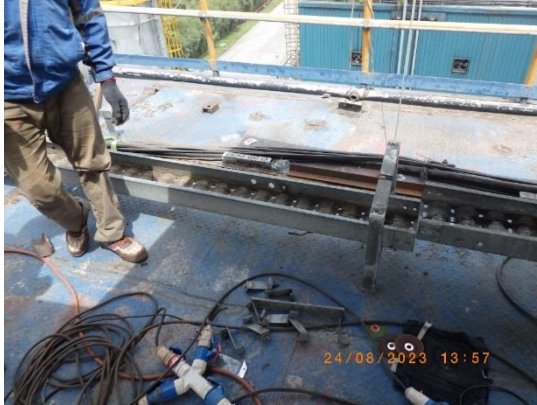
Picture 116 : Reinstalled cable tray
