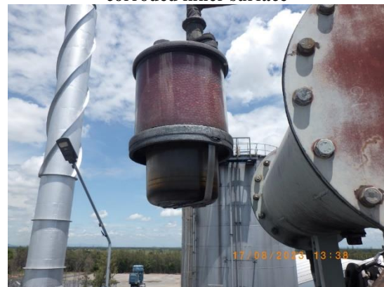
Picture 70 : Silica gel in good condition
