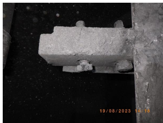
Picture 40 : Loose CE anvil bolt
