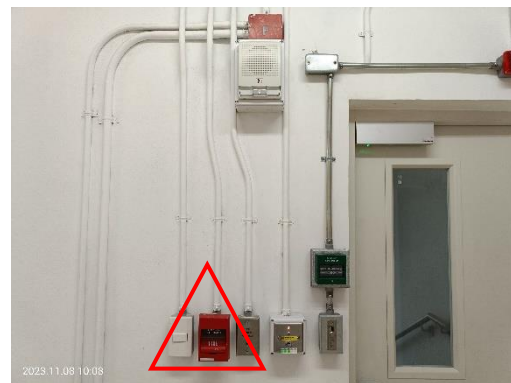
Fire Alarm Manual Station
