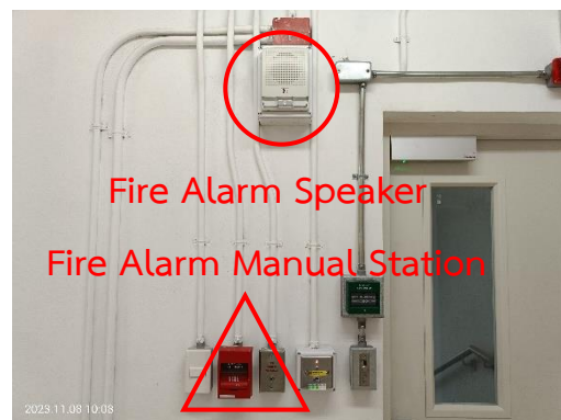
Fire Alarm Speaker & Fire Alarm Manual Station
