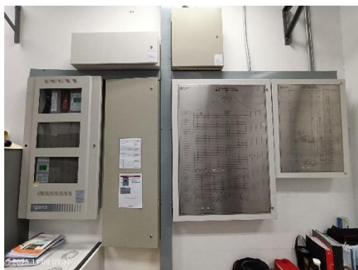
Fire Alarm Control Panel
