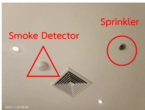
Smoke Detector & Sprinkler
