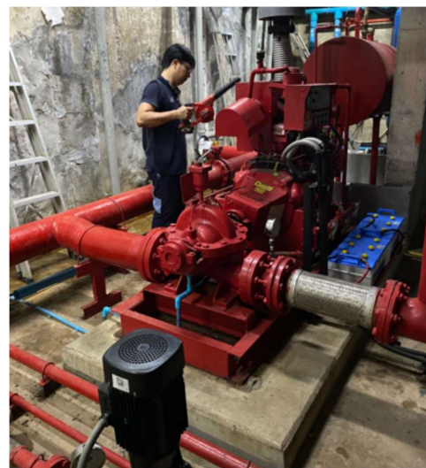
Cleaning engine fire pump
