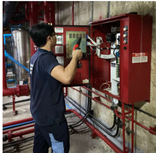
Cleaning controller fire pump
