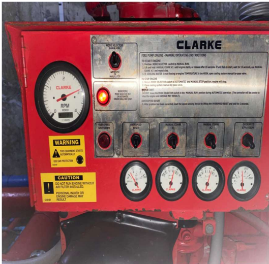
Panel engine fire pump
