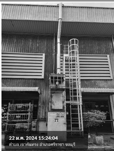
Dust Collector G.1 Forging 2
