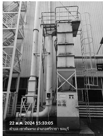
Dust Collector G.8 Forging 4
