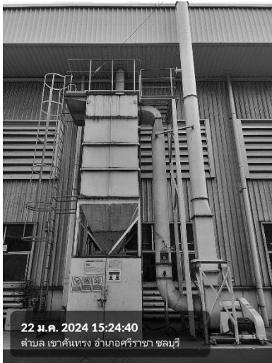
Dust Collector G.8 Forging 3
