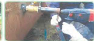
Insertion Transducer Installation
