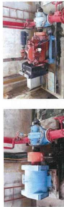
Motor Water Pumps, STP brand, Type TD12D 2969RPM, Head 102, Flow Meter 85 litres / Sec.
