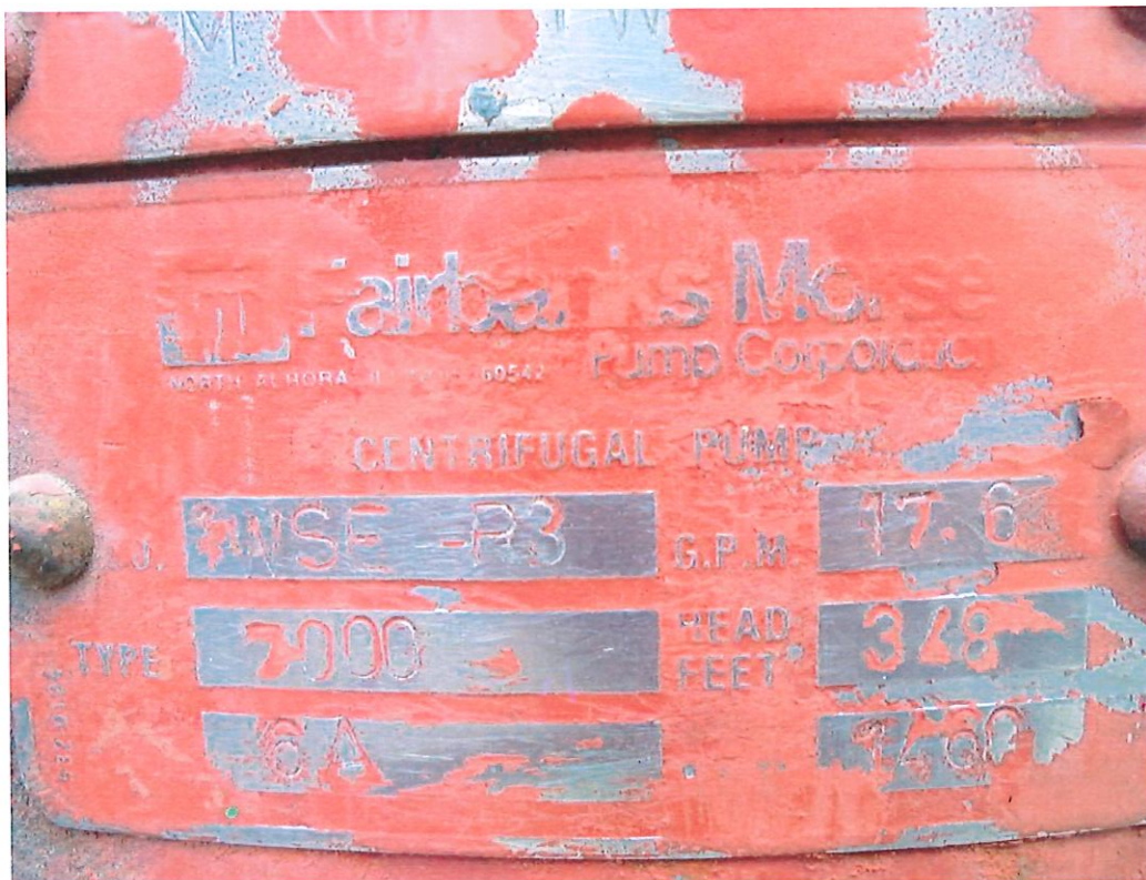
Name plate of fire water jockey pump 1WSE-P-3
