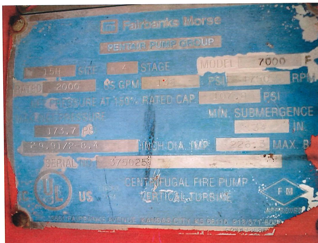
Name plate of diesel engine fire pump 1WSE-P-2
