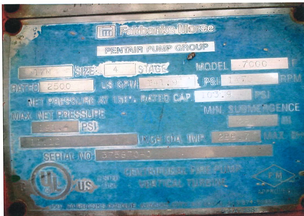
Name plate of electrical fire pump 1WSE-P-1
