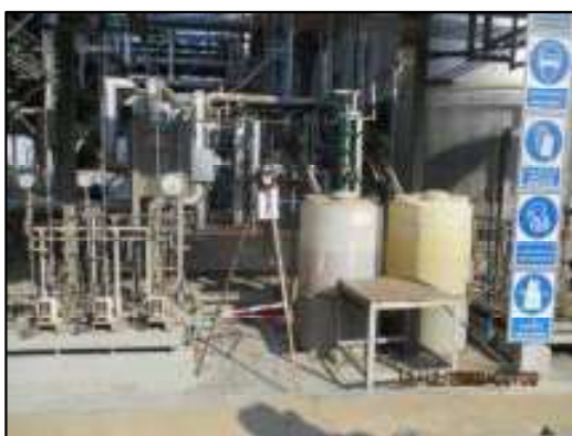
Chemical Feed pump (Phase 1)
