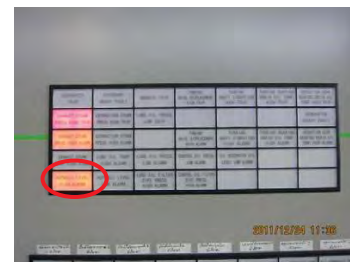
6. Level high alarm at +170mm
