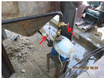
3. Check make-up water pump *Open valves
