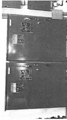
Figure 2.1 Control panel of fire pump.
