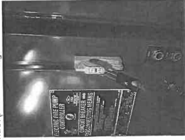
Figure 3.1 Switch on-off of control panel is damaged.
