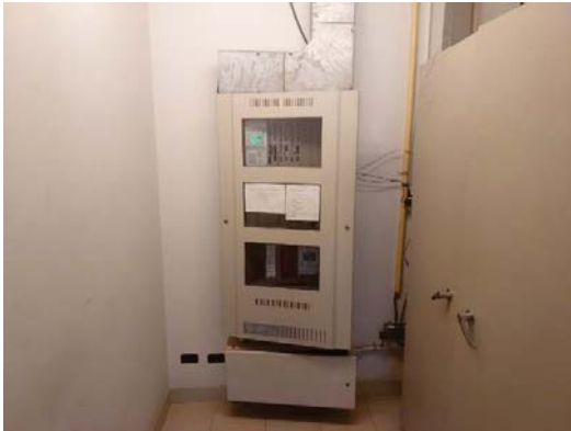
Fire Alarm Control Panel
