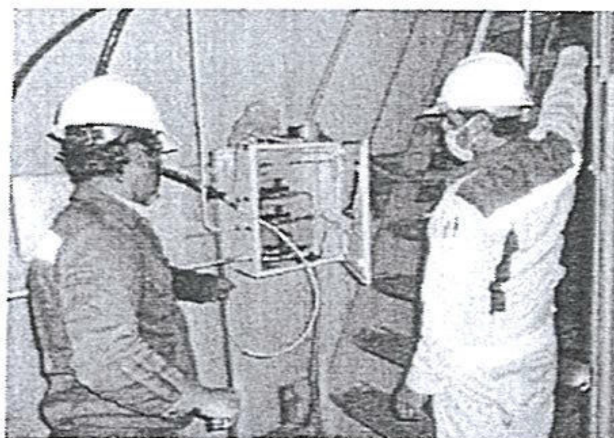
Flushing Sampling tube for Heated line stack1,2
