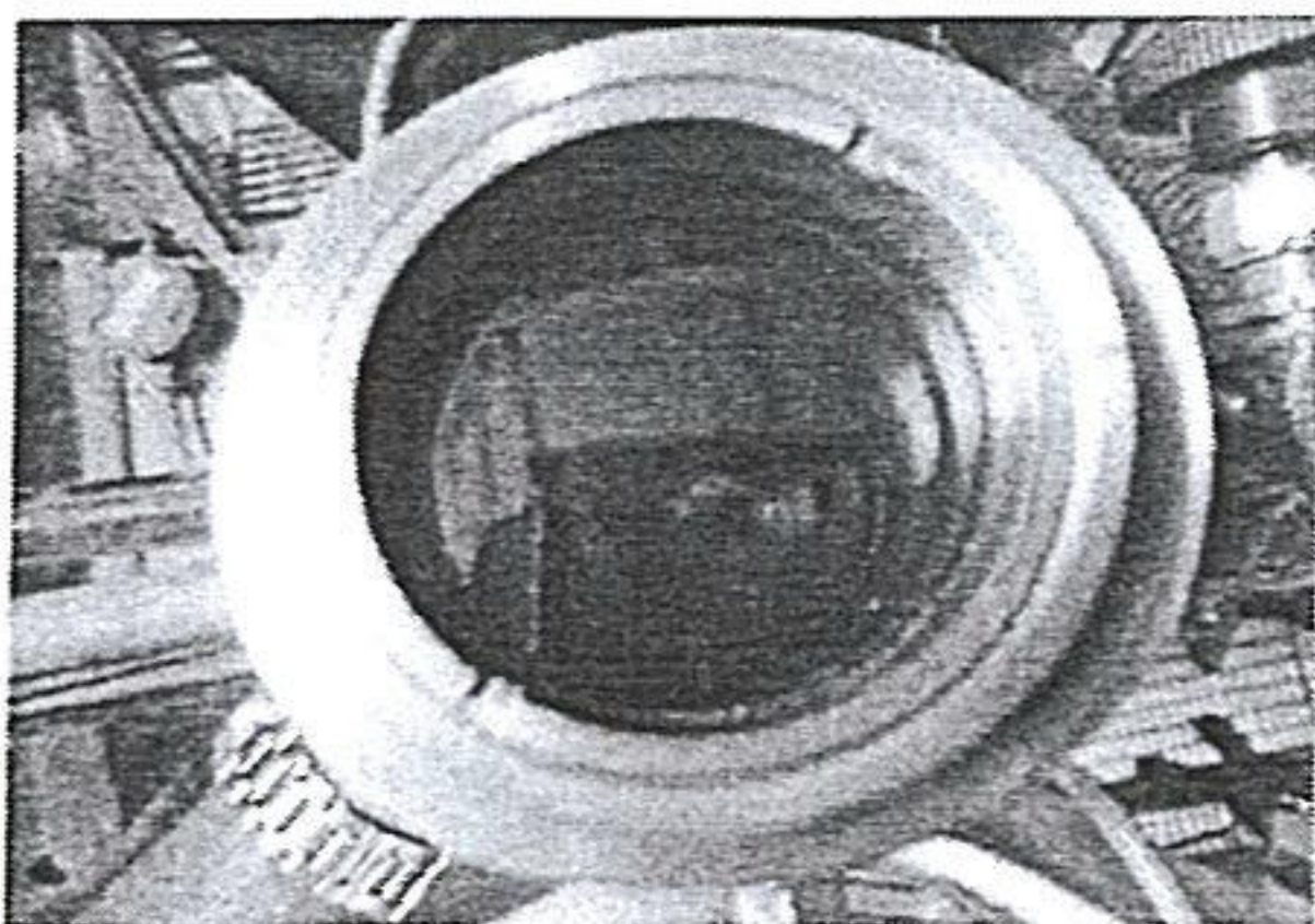
Cleaned lens for HCL sensor probe stack 2
