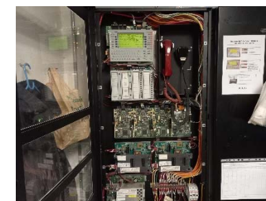
Fire Fighter Telephone System
