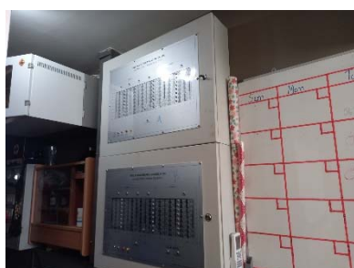
Graphic Annunciator Fire Alarm System
