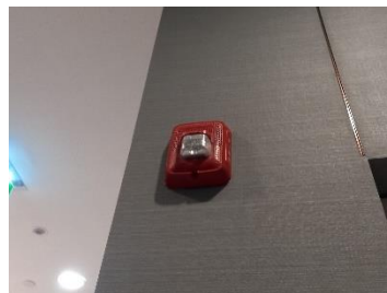
Fire Alarm Siren with Flashing Light
