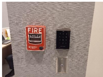
Fire Alarm Manual Station
