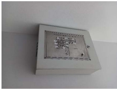
Graphic Annunciator Fire Alarm System
