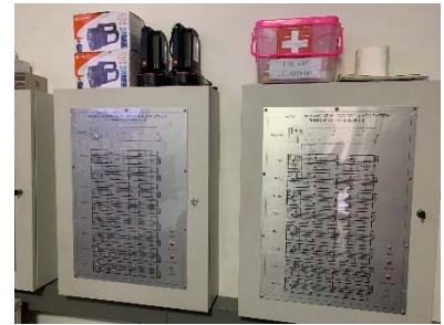
Graphic Annunciator Fire Alarm System
