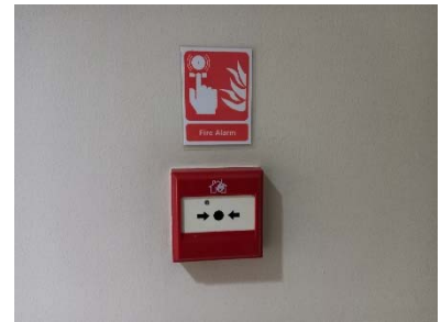
Fire Alarm Manual Station
