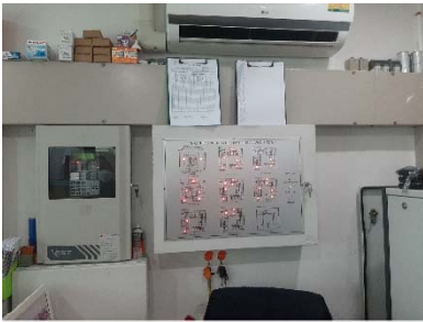
Graphic Annunciator Fire Alarm System
