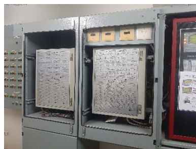
Graphic Annunciator Fire Alarm System
