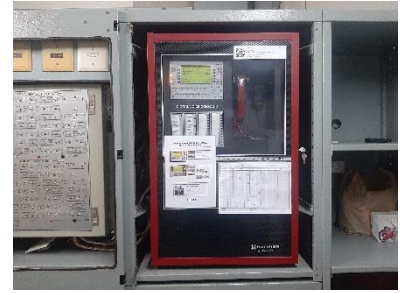
Fire Alarm Control Panel
