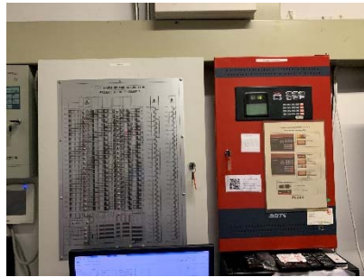
Graphic Annunciator Fire Alarm
