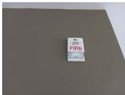
Fire Alarm Horn Strobe
