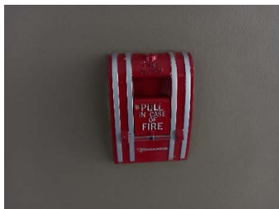
Fire Alarm Manual Station
