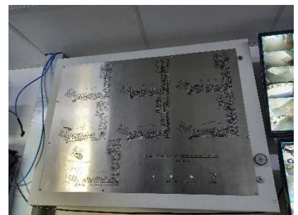
Graphic Annunciator Fire Alarm System
