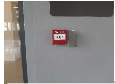
Fire Alarm Manual Station
