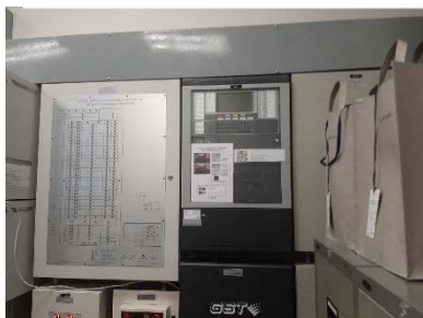
Graphic Annunciator Fire Alarm System
