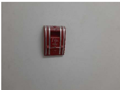
Fire Alarm Manual Station
