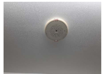
Fire Alarm Horn Strobe
