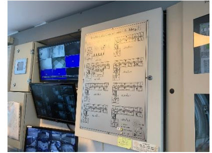
Graphic Annunciator Fire Alarm System
