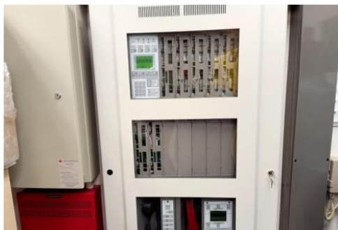
Fire Alarm Control Panel
