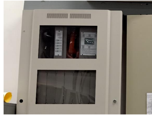
Fire Alarm Control Panel
