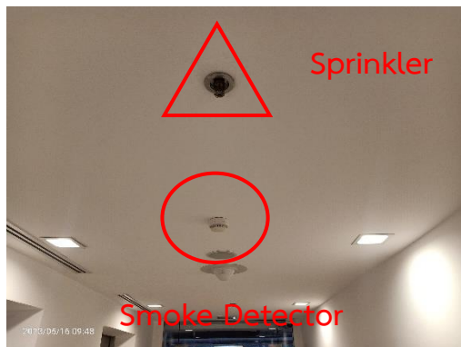
Smoke Detector & Sprinkler
