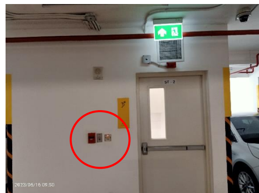
Fire Alarm Manual Station
