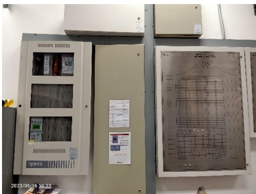
Fire Alarm Control Panel
