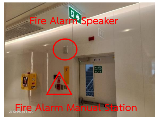
Fire Alarm Speaker & Fire Alarm Manual Station
