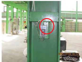
4. Start make-up water pump *Check hotwell level
