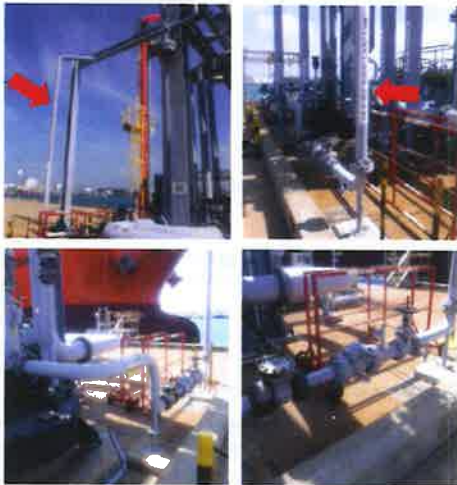
Photo4: 66D102 to ballast line still in good condition observed.
