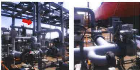
Photo5: Ballast line to 66HV130 still in good condition observed.
