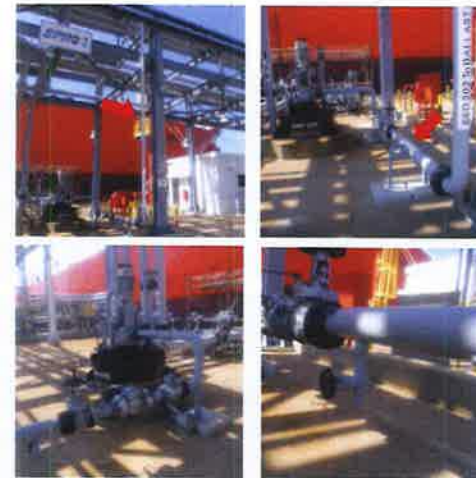
Photo6: 66D202 to ballast line still in good condition observed.
