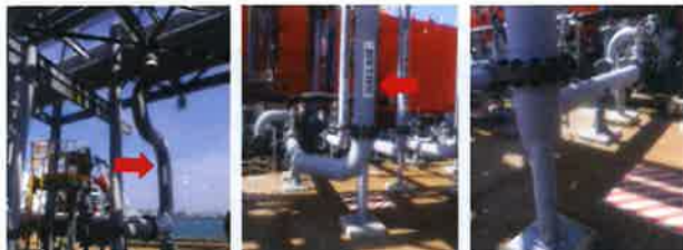
Photo9: 66K302 to ballast line still in good condition observed.
