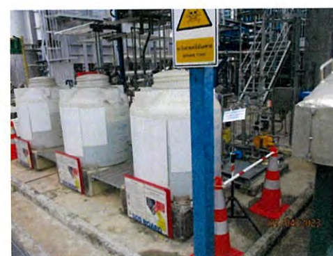
Sodium hydroxide tank (Boiler)
