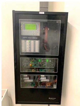
Fire alarm control panel
