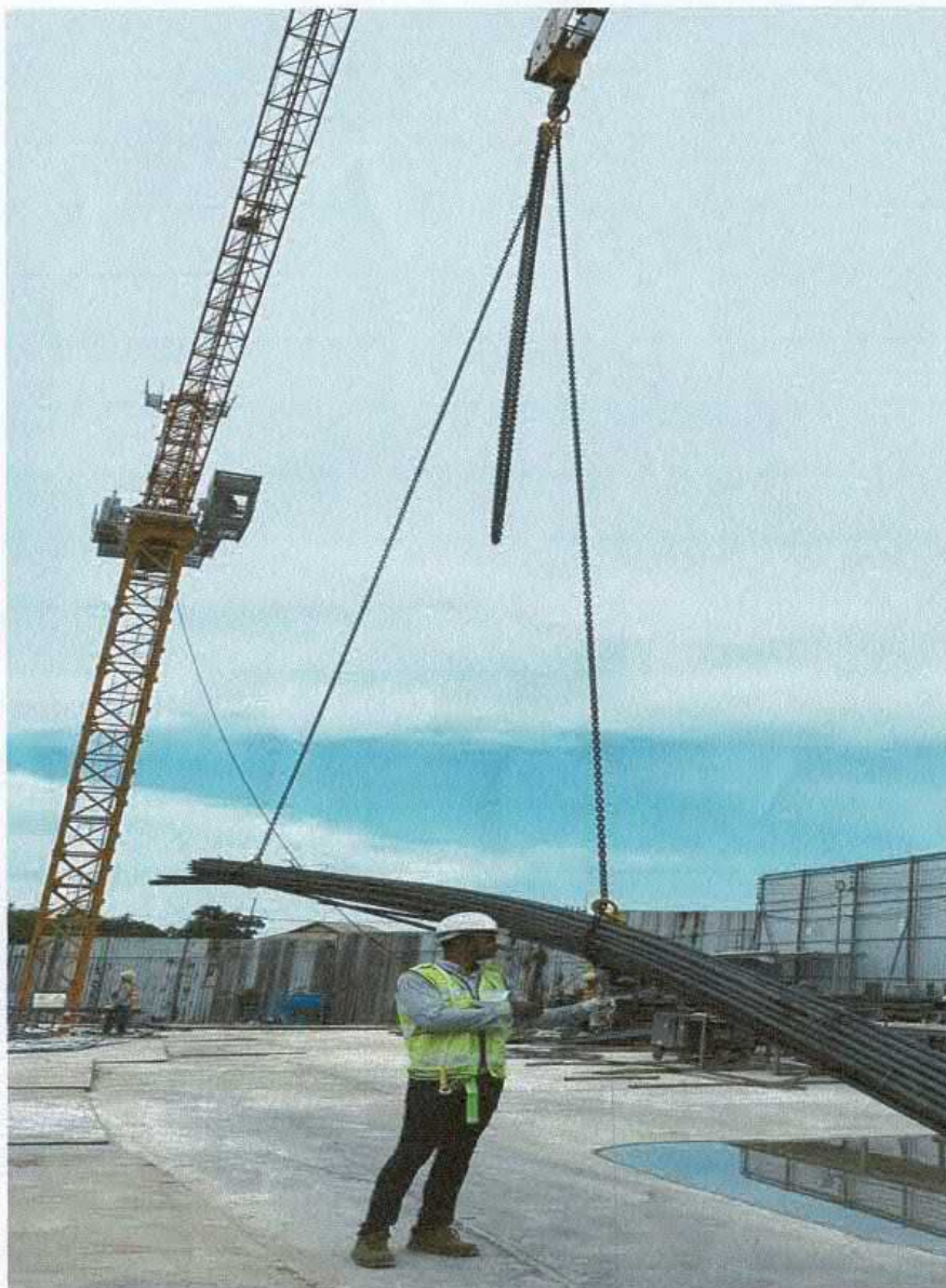
Picture : Load Test Of Tower Crane 8Ton
