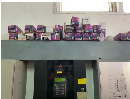
Fire Alarm Control Panel: FCP
