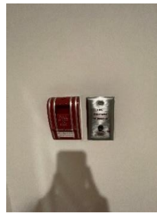
Fire Alarm Pull Station
