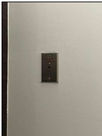
Fire Fighter Telephone Jack
