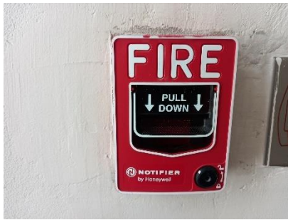
Fire Alarm Manual Station
