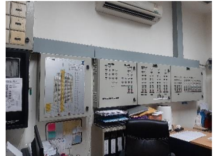
Graphic Annunciator Fire Alarm System
