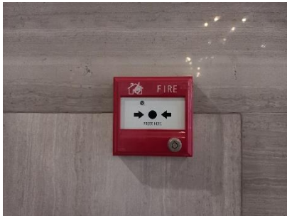
Fire Alarm Manual Station
