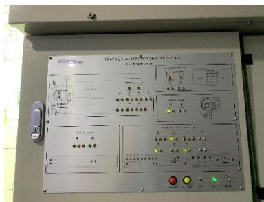
Graphic Annunciator Fire Alarm System
