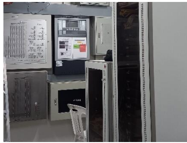
Graphic Annunciator Fire Alarm System
