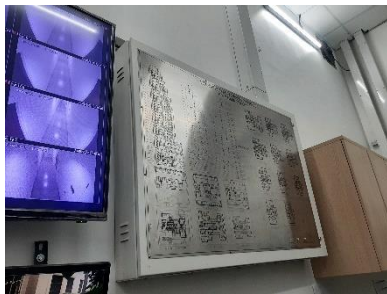
Graphic Annunciator Fire Alarm System
