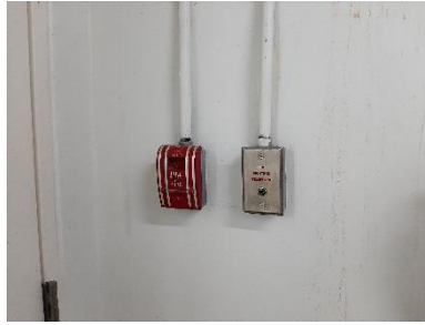
Fire Alarm Manual Station
