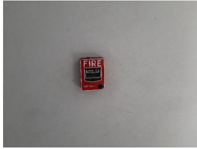
Fire Alarm Manual Station
