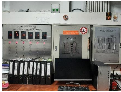
Graphic Annunciator Fire Alarm System
