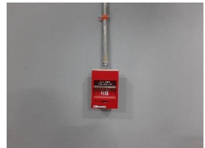
Fire Alarm Manual Station
