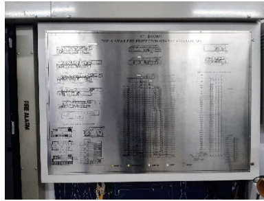
Graphic Annunciator Fire Alarm System
