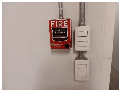
fire alarm manual station
